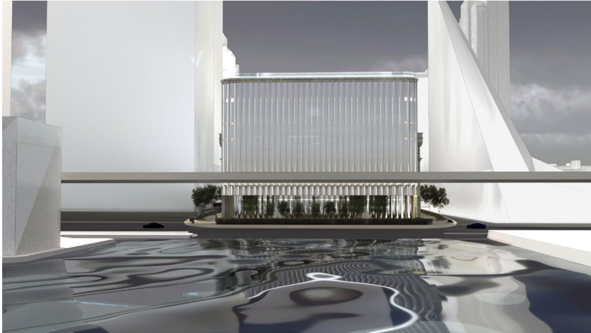
The building's façade incorporates reflective glass, angled to optimize reflectivity and positioned on the rear side to enhance natural light intake while showcasing the bathhouse to the public. This reflective surface brightens interior spaces during the day and serves as a dynamic display to engage passersby, seamlessly blending functionality with aesthetic appeal.
